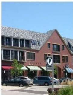
Primary Materials: Brick
