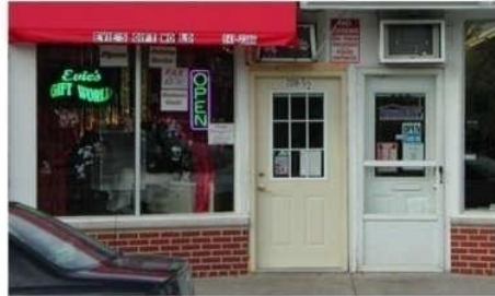
Prohibited: Residential Grade Doors on Commercial Buildings.
