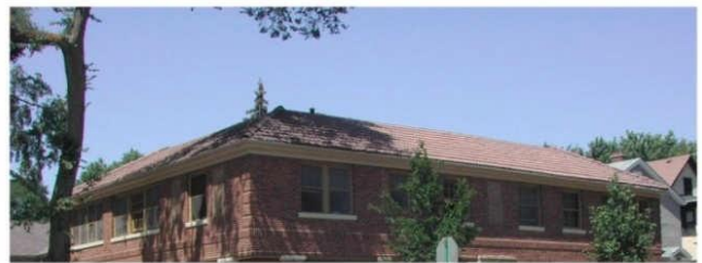
Roof Materials: Ceramic Tile
